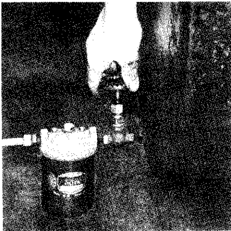
1. Check Shut-Off Valve and Line Filter. Replace or clean cartridge in line filter if dirty. Be sure to open shut-off valve.
