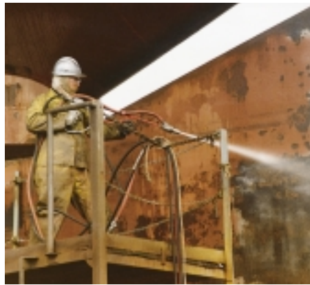
High Pressure Wet-Blasting System
