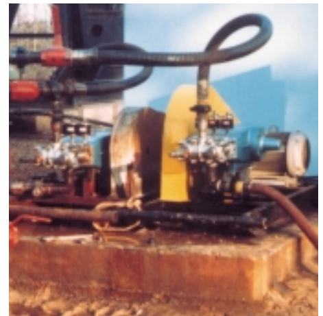
Waste-Water Re-Injection Systems
